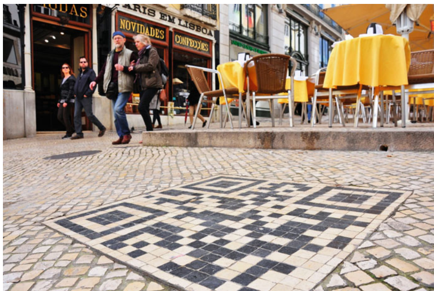
Fig. 8.2 QR codes made of compact, fine-grained, black and white Jurassic limestone cobblestones built-in in the Portuguese pavement of Lisbon for pedestrians to obtain information about historical landmarks or local history and useful city information. White cobblestones, compact, fine-grained Jurassic limestone; black stones: compact, fine-grained black Jurassic limestone. Average dimension of the cobblestones, circa 4–5 cm across
