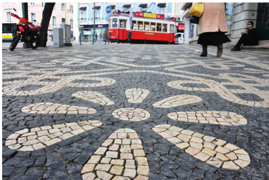
Fig. 8.1 Rosette and loop patterns in the pavement of the Duque da Terceira Square in downtown Lisbon; two examples of the many different patterns used in the typical artistic Portuguese pavement. White cobblestones, compact, fine-grained Jurassic limestone; black cobblestones, Cretaceous basalt and/or compact, fine-grained black Jurassic limestone. Average dimension of the cobblestones, circa 4–5 cm across. Note the star in the center of the rosette; it is the signature of the “ mestre calceteiro ,” the master artisan that laid that stretch of pavement
